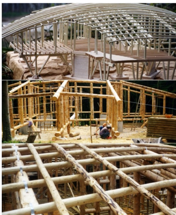
Figure 2: Model, construction and the roundwood gridshell of Westminster Lodge at Hooke Park, Dorset [7]
