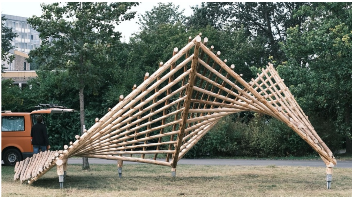
Figure 8: Realized 1:1 Hypar grid shell spanning 6 x 6 m
