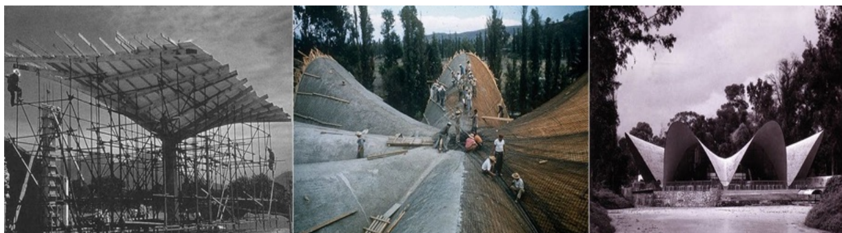
Figure 1: Félix Candela's Los Manantiales Restaurant and its timber formwork structure [4].
